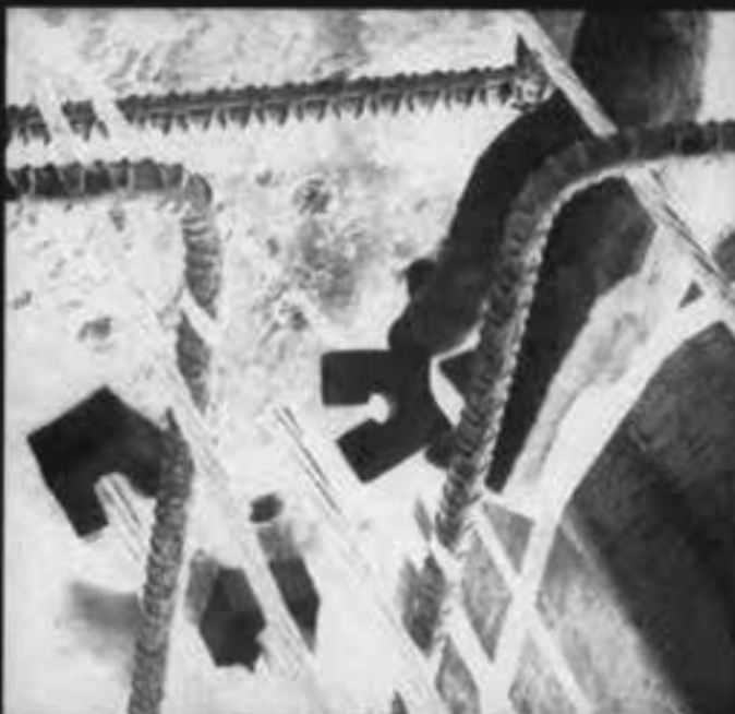
Recess Plug is easily spread open and securely attached to steel strand before concrete is poured.
