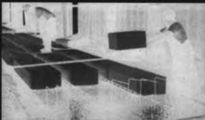
Worker places foam blockout onto fresh concrete of filigree panel. MIDSPEC DOUBLE PANEL TIE eliminates hand tied methods.
