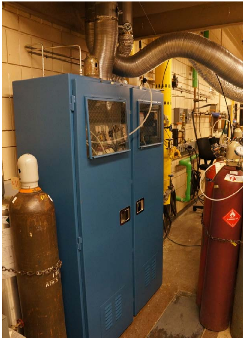
Figure 4.4 vented gas supply
