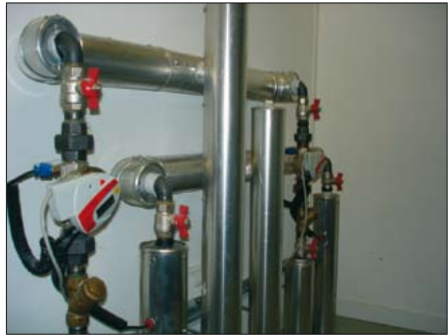
Figure 1. Heat meters with M-Bus interface and M-Bus-KNX-Gateway
