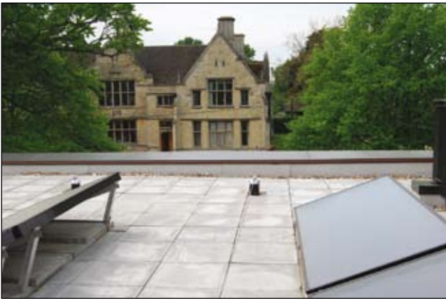
Figure 4. Sustainable resources: solar panels for the hot service water supply. Source: Andromeda
