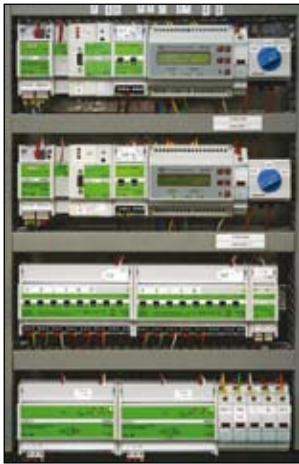
Figure 3. KNX components in the measuring room on the top floor. Source: Shäcke
