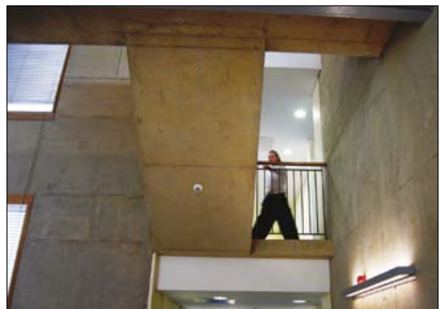
Figure 3. Energy efficiency 2: plenty of daylight and presence sensors controlling the lighting. Source: Andromeda
