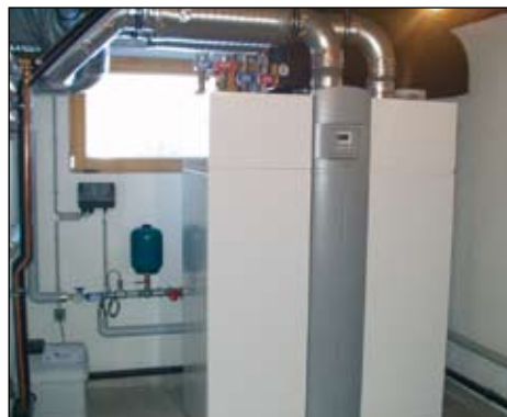
Figure 2. The integration of the air/water heat pump into the room ventilation controlled via KNX is the basis for the low energy demand
