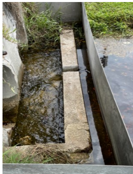
The weir after being cut by workers for the City of Melbourne.
